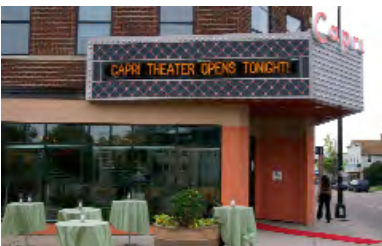
The marquee has been retrofitted with new electronic reader boards and LED light bulbs.
